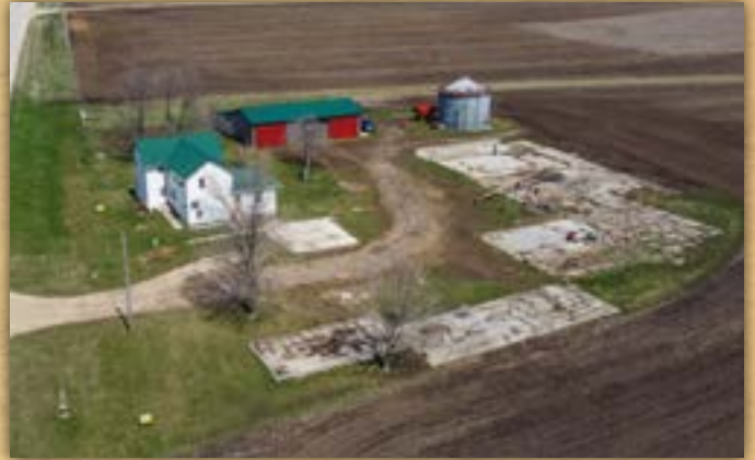
Acreege, looking north, northeast
