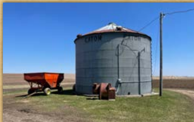
Grain bin, looking east
