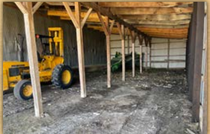
Machine shed, looking west (Open bays of north lean-to shed)
